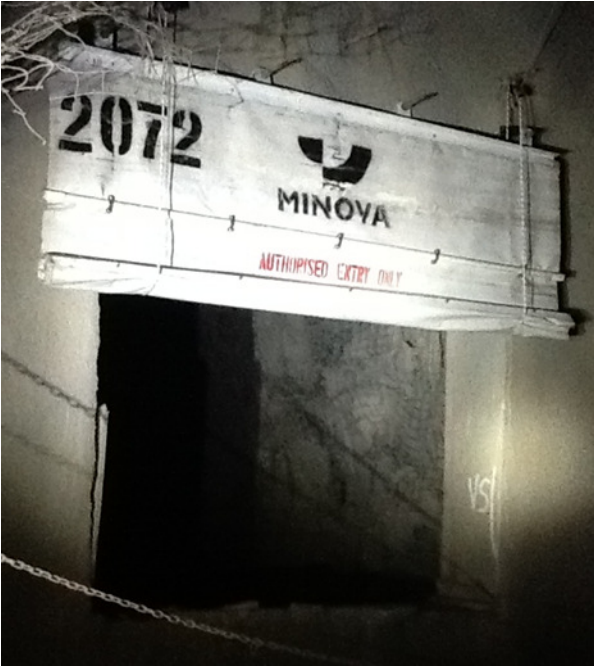
FIG 7 - An installed Strengthened QBC with the integrated stop log (MIM, 2014)
